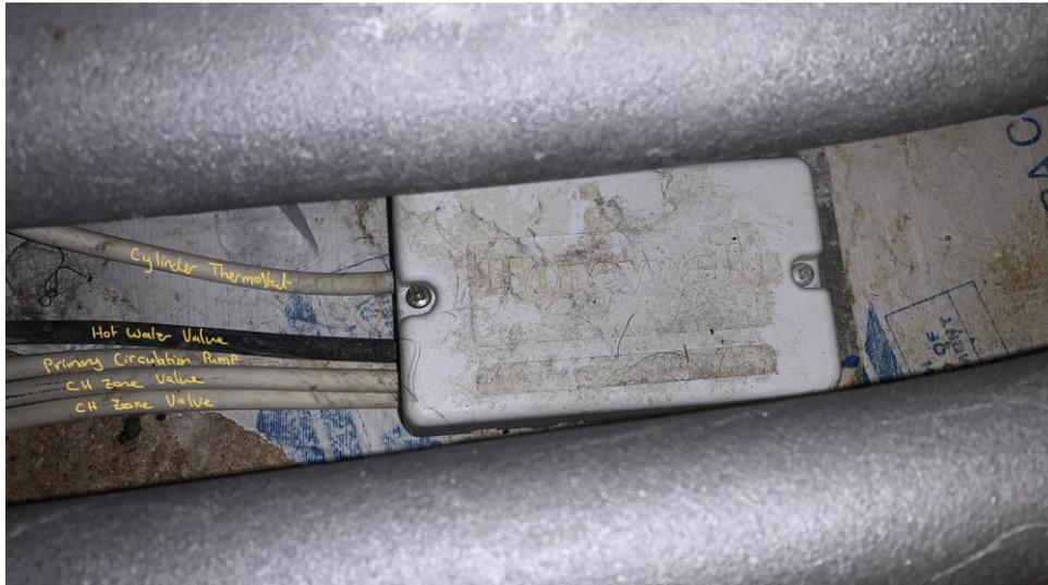
The interior is a lot messier than the wiring diagrams shown above, and unfortunately does not confirm to the same block numbering as in the diagrams. What I have done is, through mapping back the connections from the zone valves, pump and cylinder stat, and my expectation of the number of wires coming to terminal blocks, I have done my best to interpret the wiring. In the photo below I have written on the connections relative to the number in the wiring diagram to try and make sense of it.
