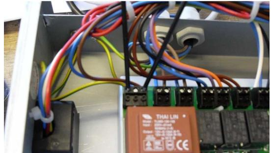
5. With the power off, check for continuity from the pressure switch. Measure between the nearest pin to the front of the burner plug and the black wire on the burner terminal of the PCB.
