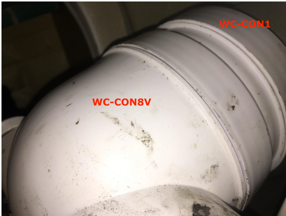
How the two connectors are fitted
